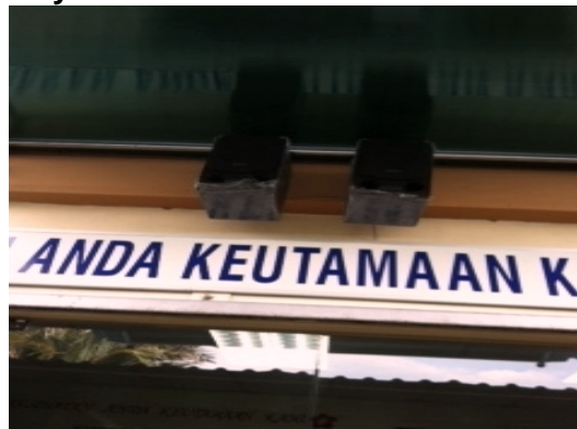
After installation of speaker
