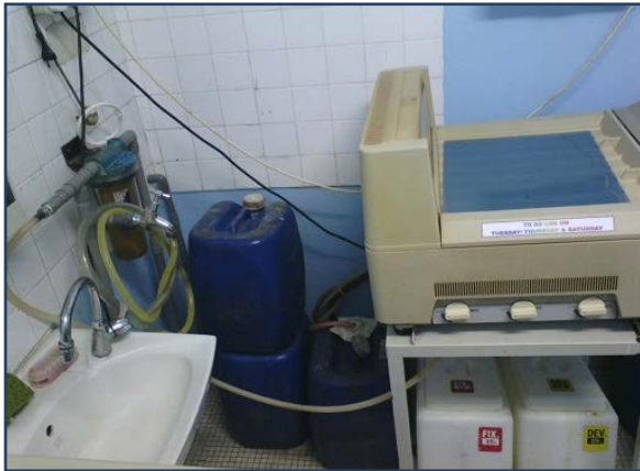
Picture: Before the installation of UPVC pipe, all chemical tank stored in dark room and produce ammonia odour.
