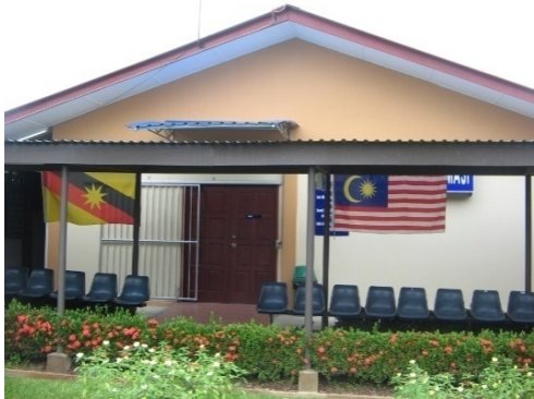
Before installation of speaker
